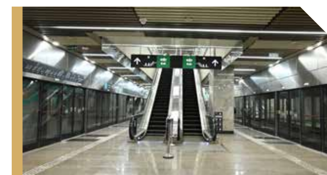
MUMBAI METRO LINE
