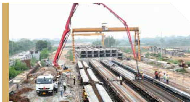
DWARKA CASTING YARD
