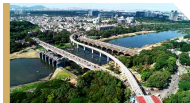
PUNE ELEVATED METRO
