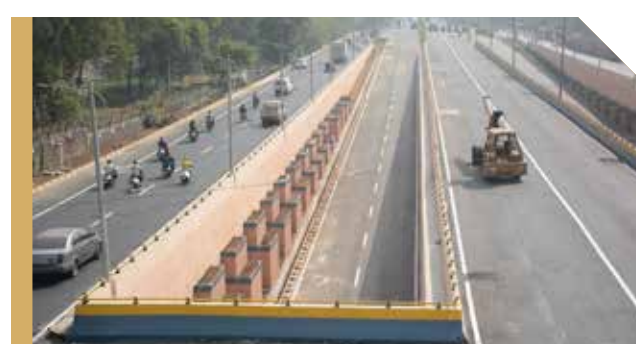
KSB UNDERPASS PUNE
