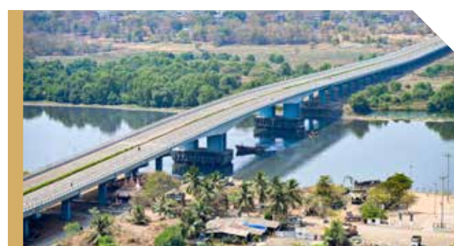
MOTHGOAN CREEK BRIDGE
