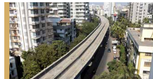
MUMBAI METRO LINE
