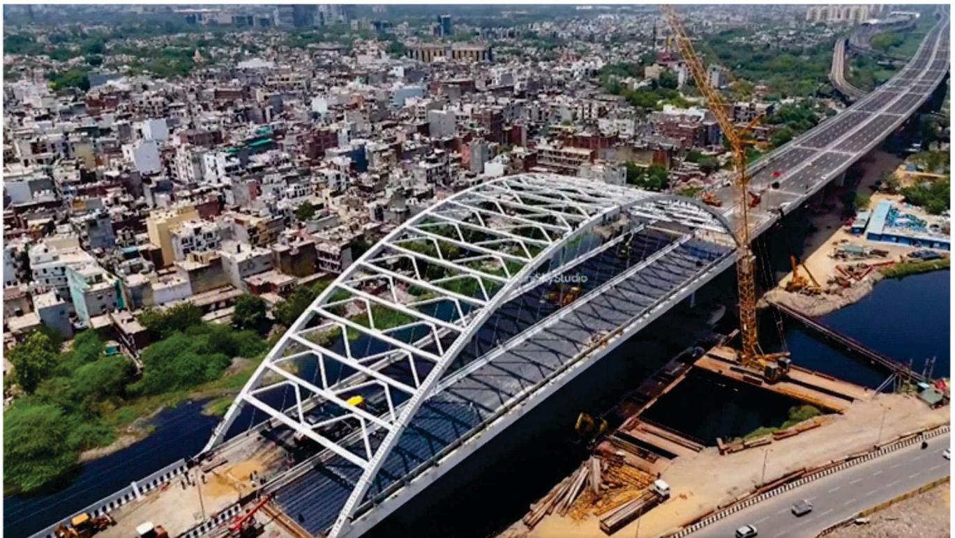
Network Arch Bridge project in New Delhi.
