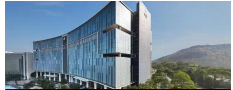
Embassy TechZone Pune (5.5 msf)
