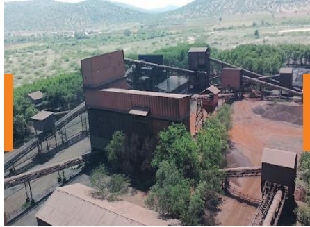
Ananthapur Unit-II Andhra Pradesh
